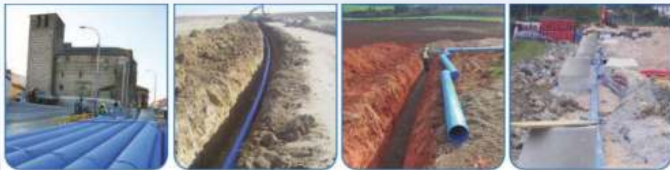
Picture 2: PVC-BO pipes for the transport of drinking water, for the supply of urban and industrial areas, and for filling reservoirs and dams.
