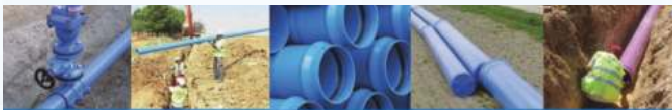
Picture 1: Installation of PCV-BO Pipes
